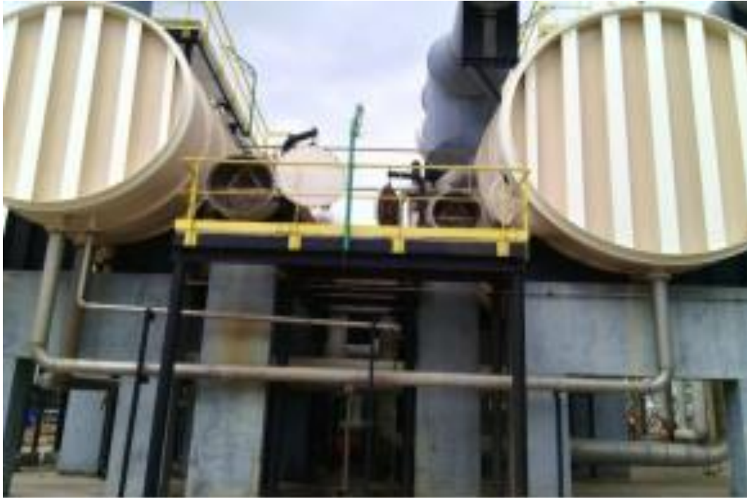
Figure III.6: Des tubes U prise de la station de dessalement TCD 6-8000 [78].
