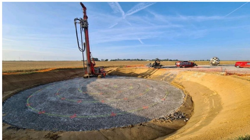
Figure.II.4. Vibro compactage. [Menard France]
