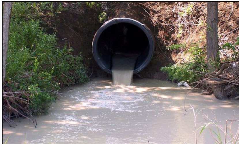
Figure 7: Sewage outfalls in valleys [68]
